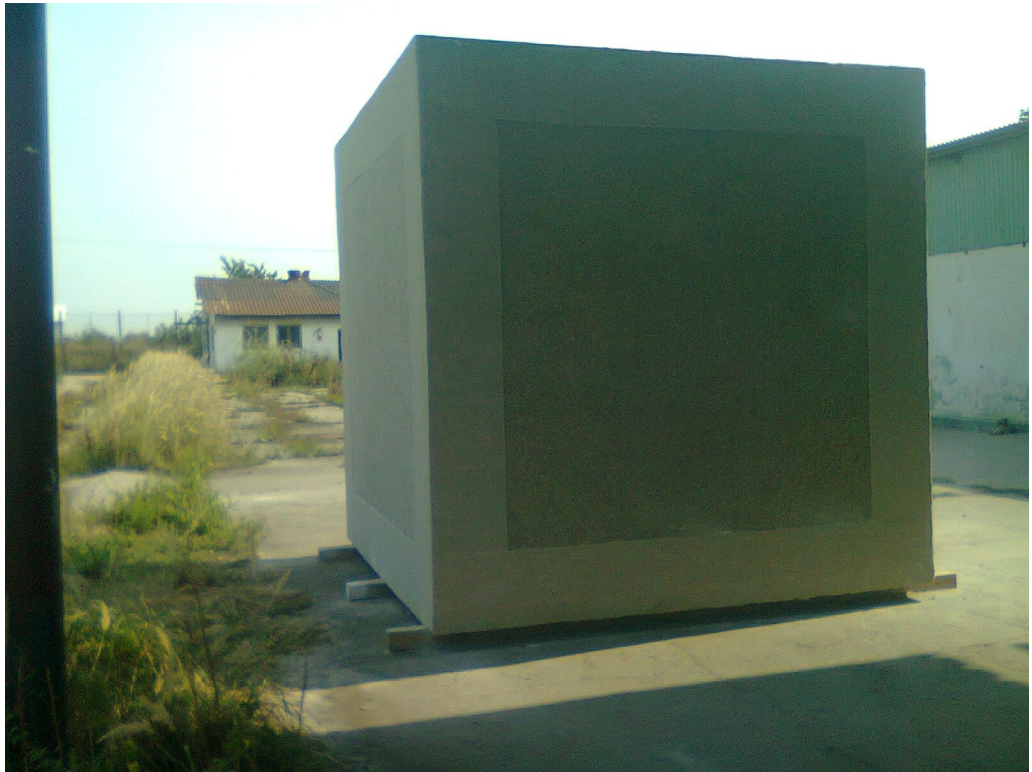
Fig.24. Construction (dimensions 3x3x3 m). Exterior 2
