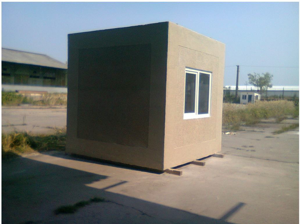
Fig.25 Construction (dimensions 3x3x3 m). Exterior 3
