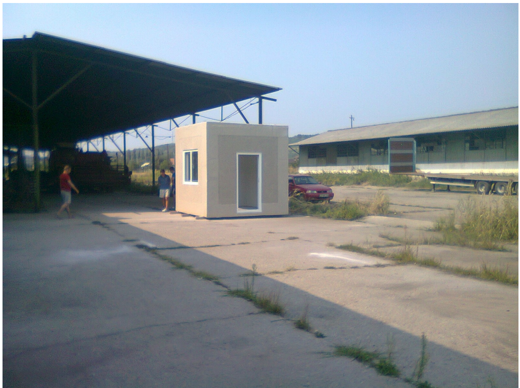
Fig.23. Construction (dimensions 3x3x3 m). Exterior 1
